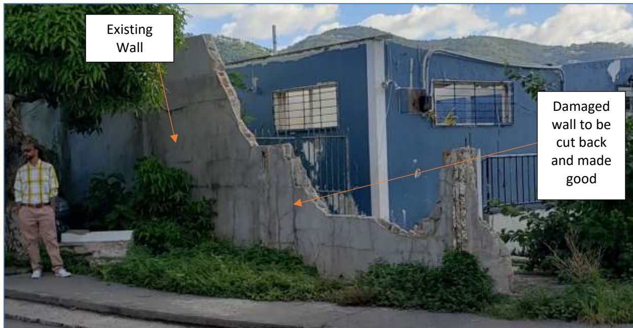
Figure 2 - Photograph of existing damaged walls to be cut back and made good.
