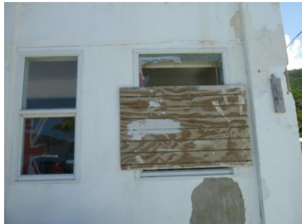
PHOTO 5: JVD ADMIN BUILDING BEFORE CONSTRUCTION 2
