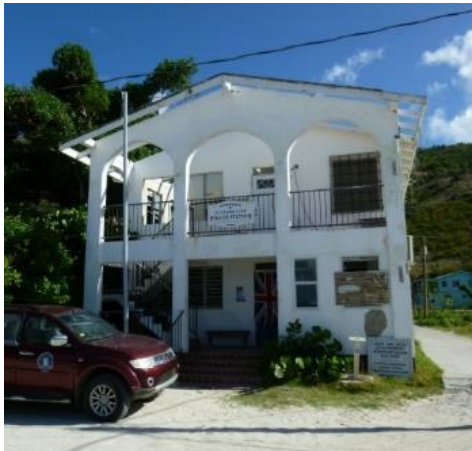
PHOTO 6: JVD ADMIN BUILDING BEFORE CONSTRUCTION 1
