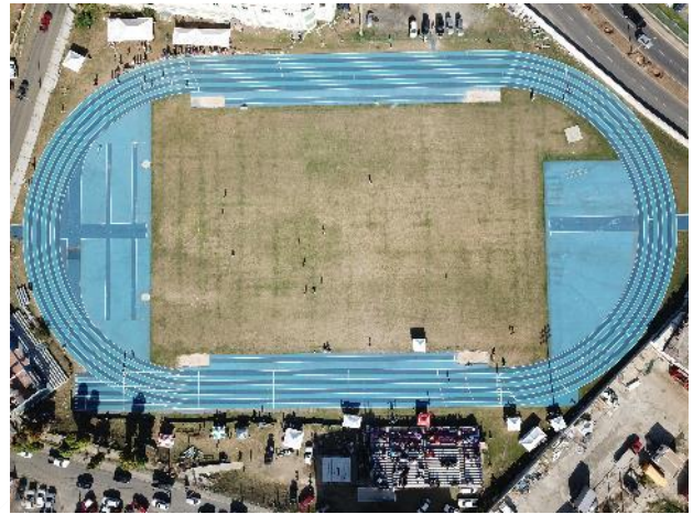
PHOTO 3: TRACK AFTER CONSTRUCTION 2
