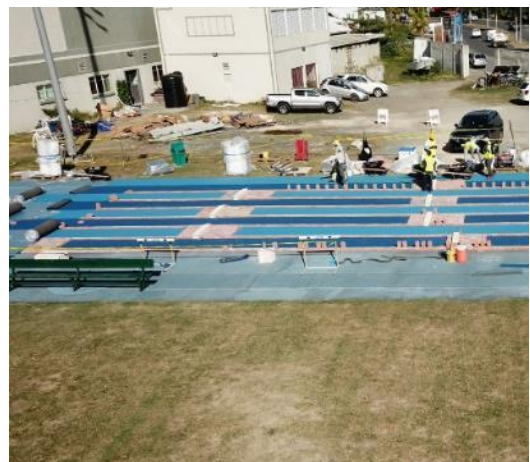
PHOTO 1: TRACK DURING CONSTRUCTION
