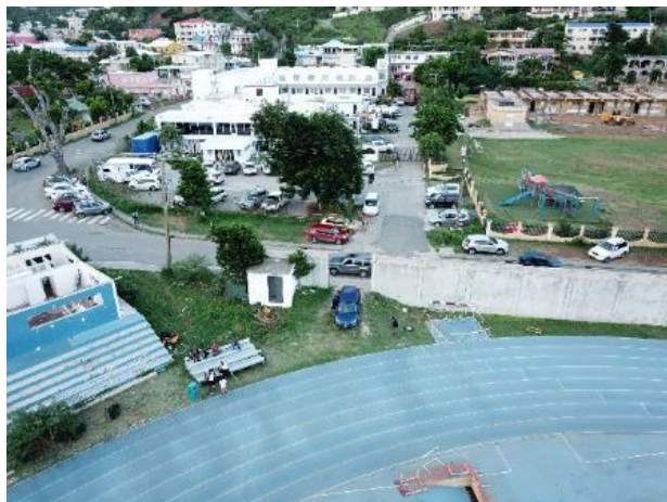
PHOTO 2: TRACK BEFORE CONSTRUCTION
