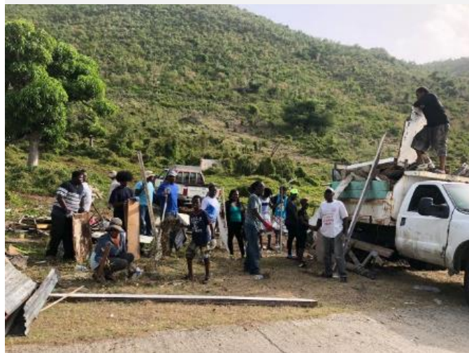
PHOTO 9: A TEAM ASSISTING DEBRIS CLEARANCE, AUGUST 2018
