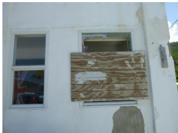
PHOTO 5: JVD ADMIN BUILDING BEFORE CONSTRUCTION 2
