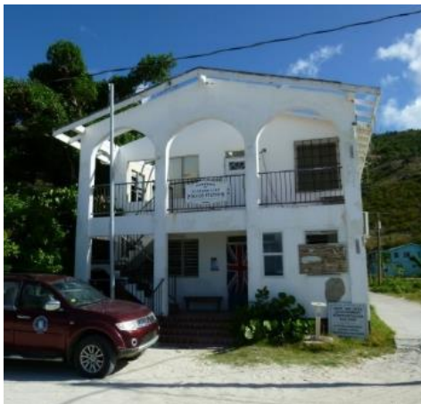
PHOTO 6: JVD ADMIN BUILDING BEFORE CONSTRUCTION 1
