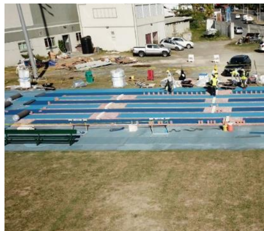
PHOTO 1: TRACK DURING CONSTRUCTION
