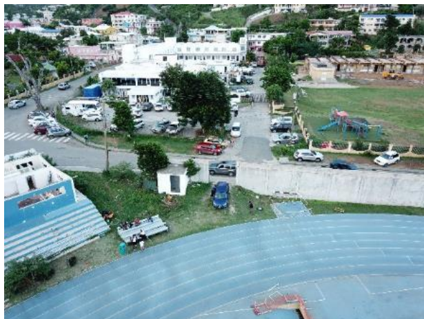
PHOTO 2: TRACK BEFORE CONSTRUCTION
