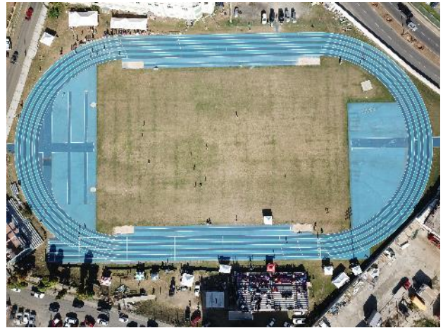
PHOTO 3: TRACK AFTER CONSTRUCTION 2
