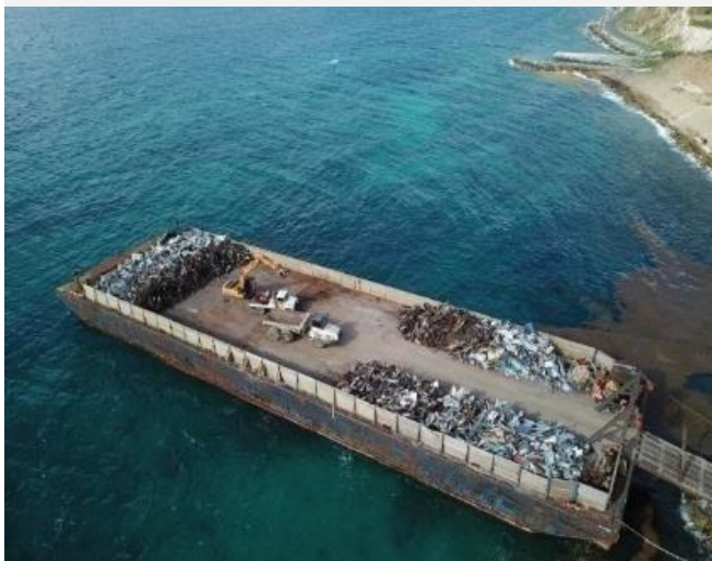
PHOTO 10: BARGE DURING THE DEBRIS CLEARANCE IN AUGUST 2018
