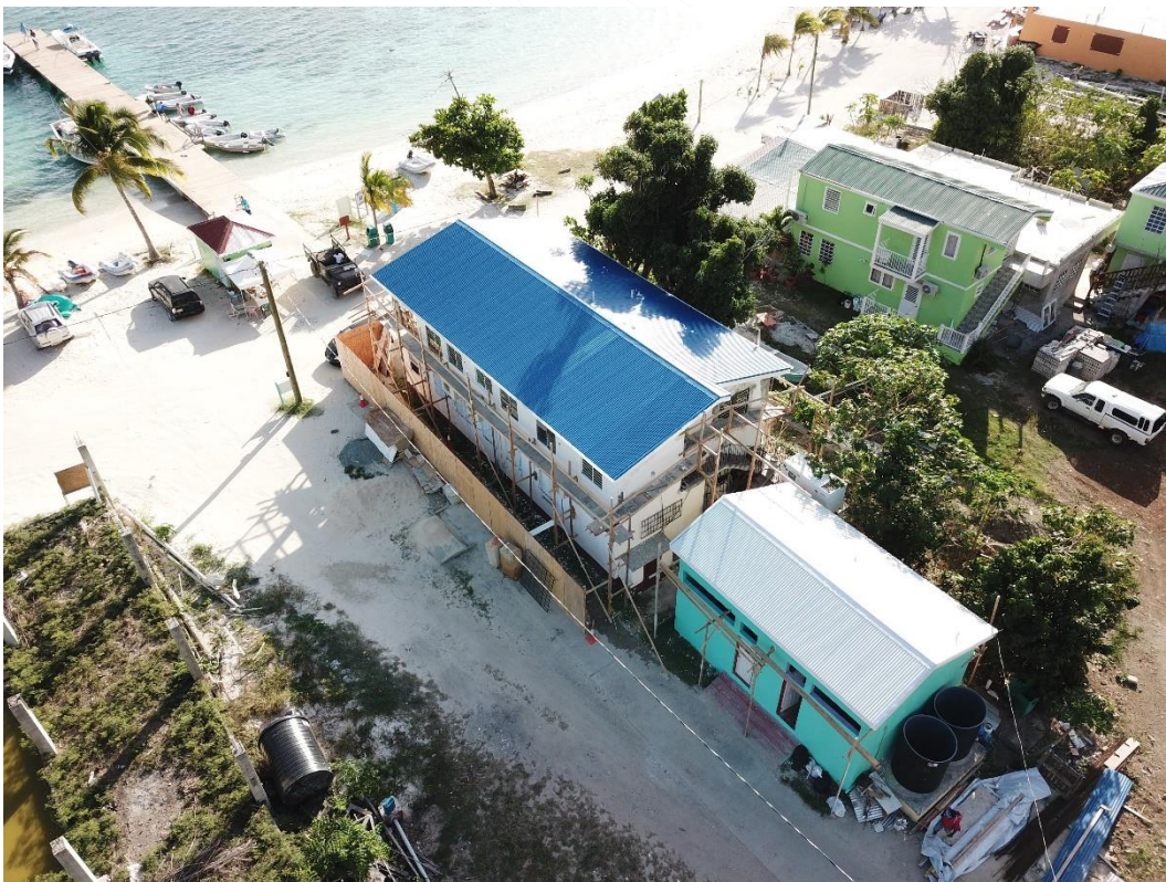
PHOTO 7: CONSTRUCTION OF NEW ROOF OF JVD ADMIN BUILDING
