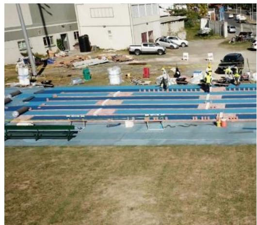
PHOTO 1: TRACK DURING CONSTRUCTION
