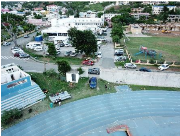
PHOTO 2: TRACK BEFORE CONSTRUCTION
