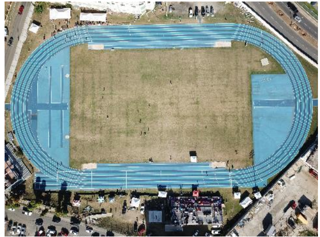
PHOTO 3: TRACK AFTER CONSTRUCTION 2
