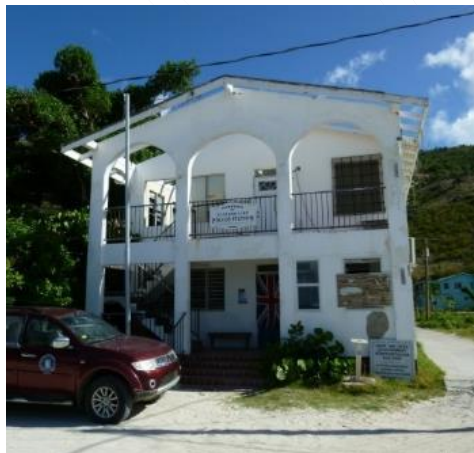
PHOTO 6: JVD ADMIN BUILDING BEFORE CONSTRUCTION 1
