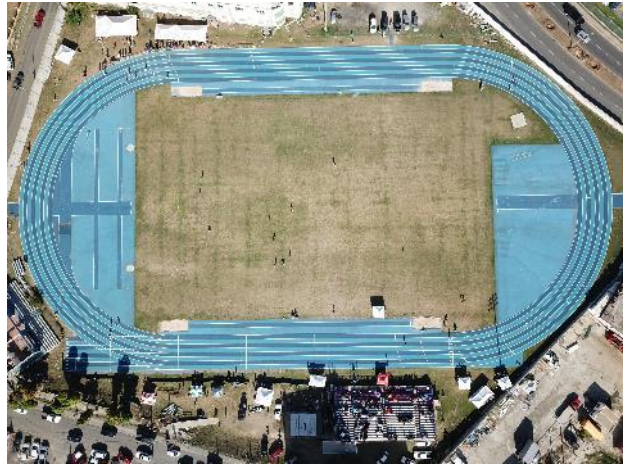
PHOTO 3: TRACK AFTER CONSTRUCTION 2
