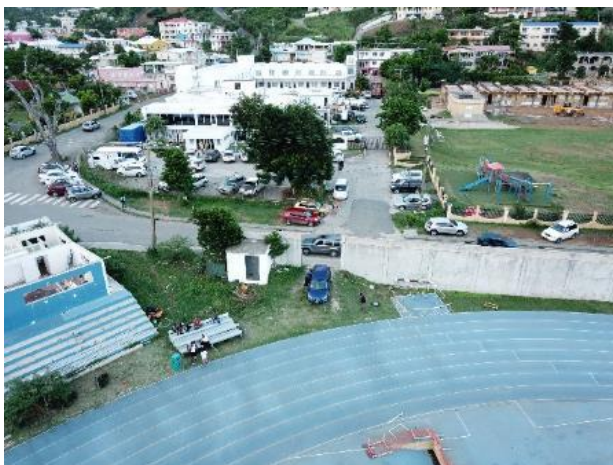
PHOTO 2: TRACK BEFORE CONSTRUCTION
