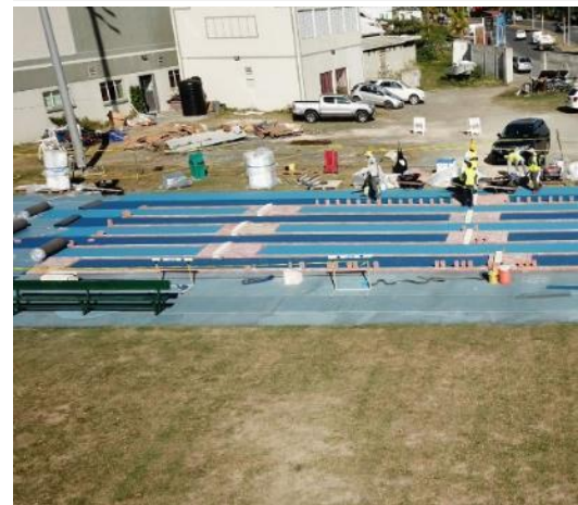
PHOTO 1: TRACK UNDER CONSTRUCTION
