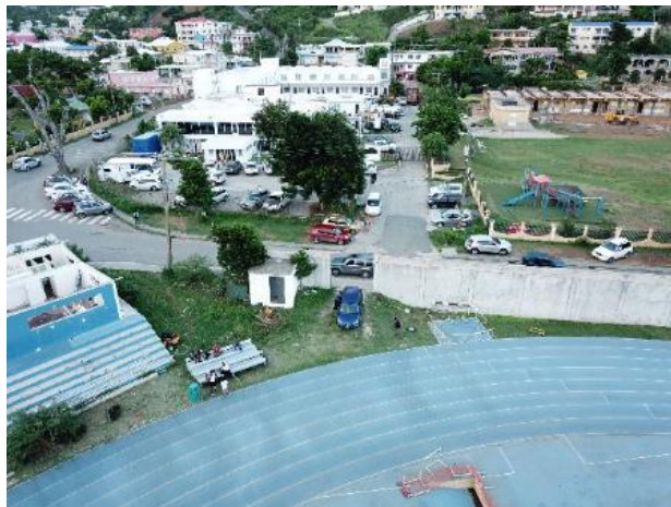
PHOTO 2: TRACK BEFORE CONSTRUCTION
