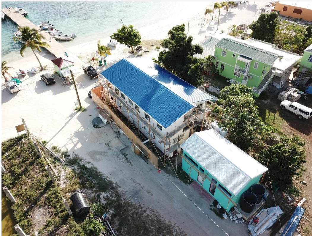
PHOTO 8: CONSTRUCTION OF NEW ROOF OF JVD ADMIN BUILDING
