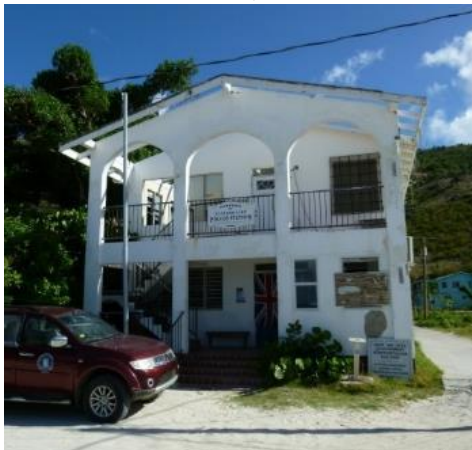
PHOTO 6: JVD ADMIN BUILDING BEFORE CONSTRUCTION 1
