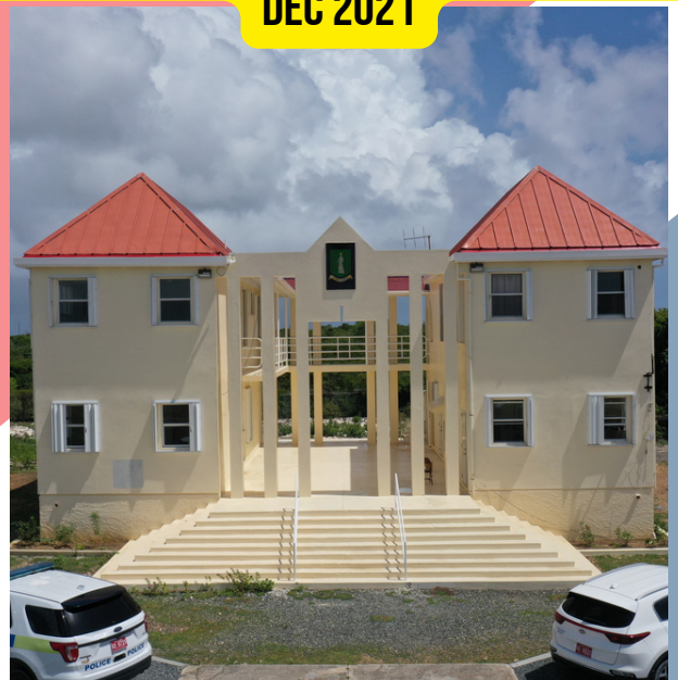
THEODOLPH FAULKNER ADMINISTRATION BUILDING DEC 2021
