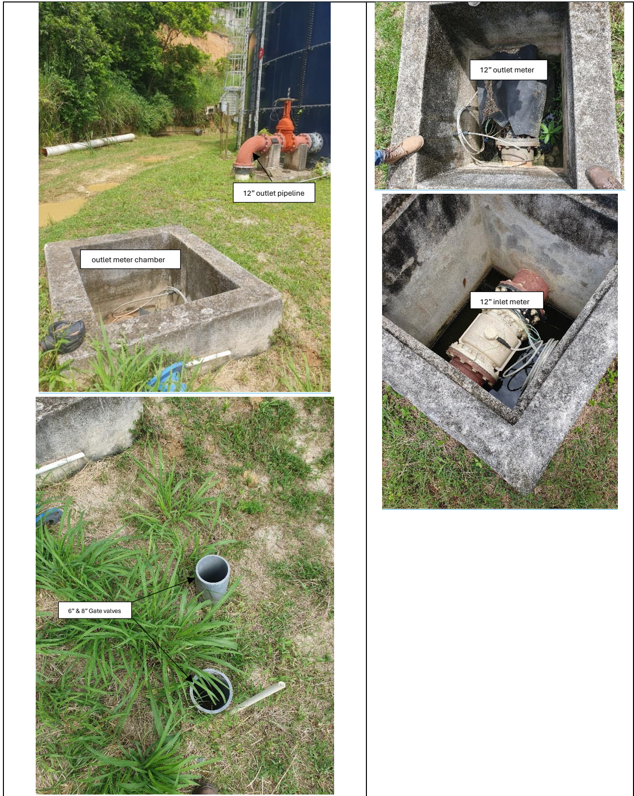
Photo 5a: Sabbath Hill Reservoir
