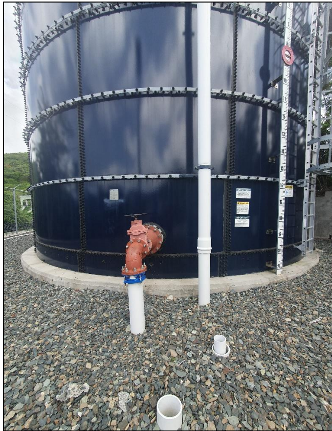
Photo 4: Zion Hill Reservoir
